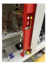
The electrical panel that contains the compressor frequency converters features a forced convection heat transfer. The boxes are equipped with special metal sheet labyrinth plates to prevent dust or snow suction.
